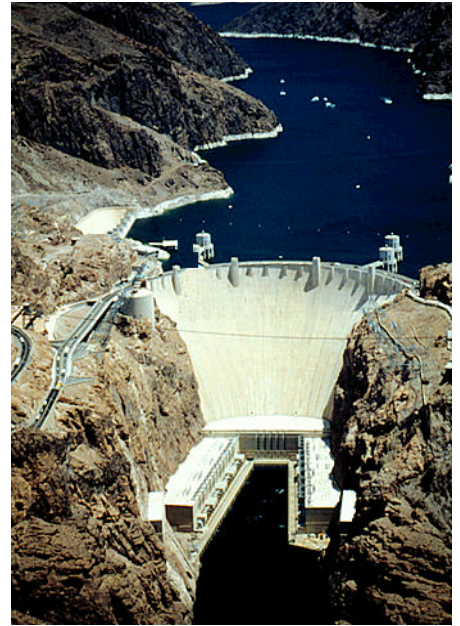
Figure 143: Barrage ou route ?
